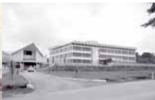
Wisma Putra Building 1966 -2001 Bukit Petaling, Kuala Lumpur.
