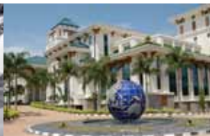
Wisma Putra Complex 2001 - Present Putrajaya
