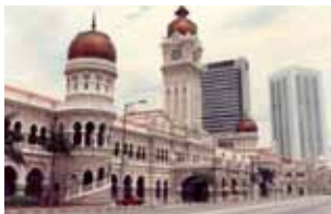
Federal Secretariat 1956 -1966 Sultan Abdul Samad Building, Kuala Lumpur.
